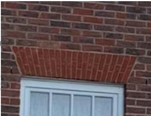
Flat segmental red brick arches
