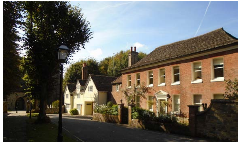
Horsham Stone Slate roofs within Causeway
