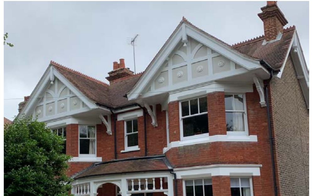
Timber sliding sash windows
