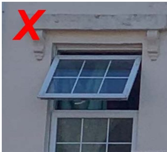
The use of plastic windows do not reflect the character of the conservation area, this is particularly evident in the lack of detailing and the changes to opening mechanisms.
