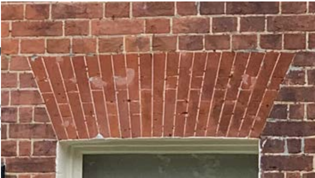
Flat segmental red brick arches
