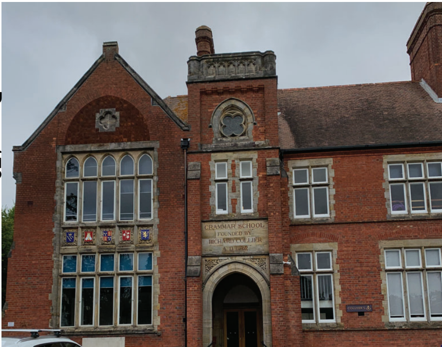
Grade 2 listed building used as a sixth form college (The College of Richard Collyer)
