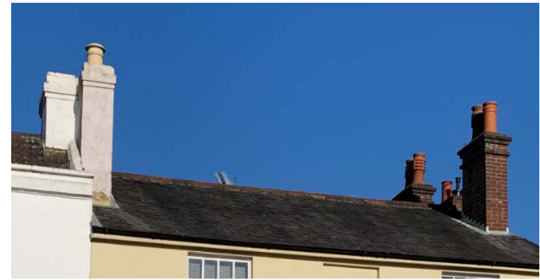
Variation of chimneys within the conservation area
