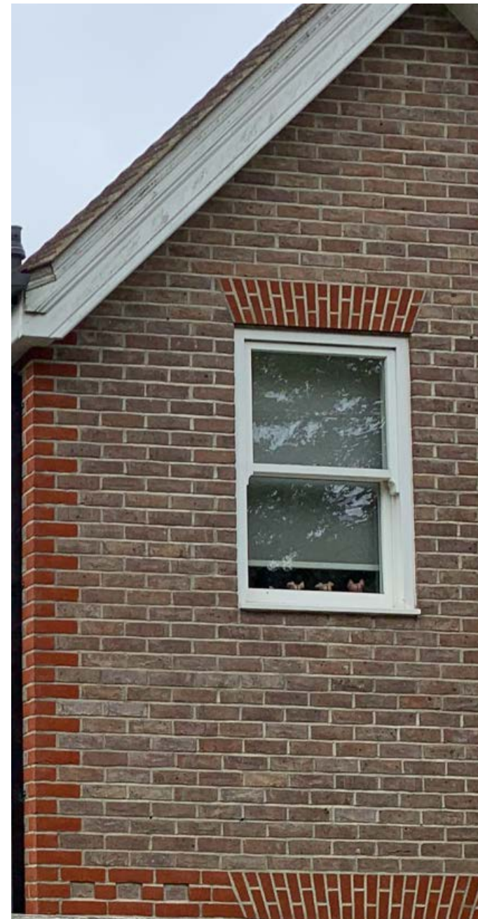
Modern stretcher bond with modern interpretation of quoin and header detailing.
