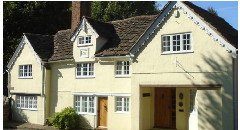
Horsham Stone slate roof
