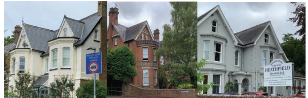
Images 2 - 4 show the locally listed buildings of 84, 86 and 88 Hurst Road. These are described within the Horsham Town Local List and would be considered to be non-designated heritage assets. Image 2 - 84 Hurst Road "Two and a half storey detached formed house. Painted render with slate roof. Two identical bay windows and central porch: modern extension to east. Group value with 23, 25, 84 & 86 Hurst Road. c.1890. Image 3 - 84 Hurst Road "Large house facing on to Hurst Road. Double fronted, two and a half storeys. Large bay windows in rendered façade with slate roof over. One large and one smaller gable with decorated barge boards. Group value with 23, 25, 86 and 88 Hurst Road. c.1890. Image 4 - 88 Hurst Road "Two and a half storey detached formed house. Painted render with slate roof. Two identical bay windows and central porch: modern extension to east. Group value with 23, 25, 84 & 86 Hurst Road. c.1890"
