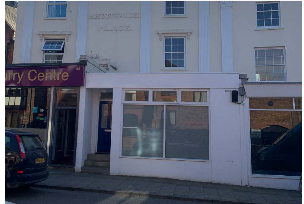
The properties within Brunswick Place have been extended to provide additional commercial space. Whilst the extensions may contribute to the historic narrative of the buildings they do not reflect the original polite appearance of the terrace.
