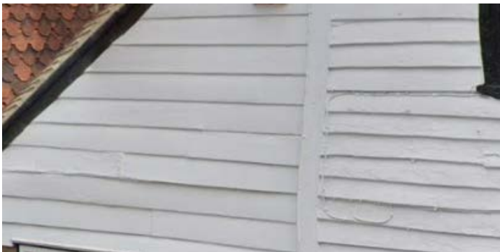
Differences between modern and traditional weatherboarding
