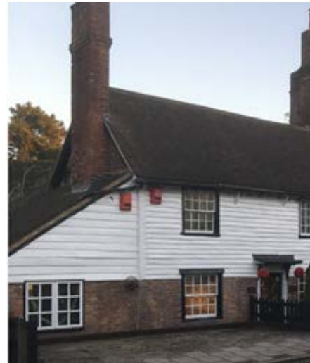
46 London Road timber framed cottage
