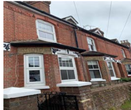
Above can be seen the terrace of Victorian properties set back slightly from the road with small front gardens. The detailing of the terrace can be seen below with decorative details above the windows and doors.
